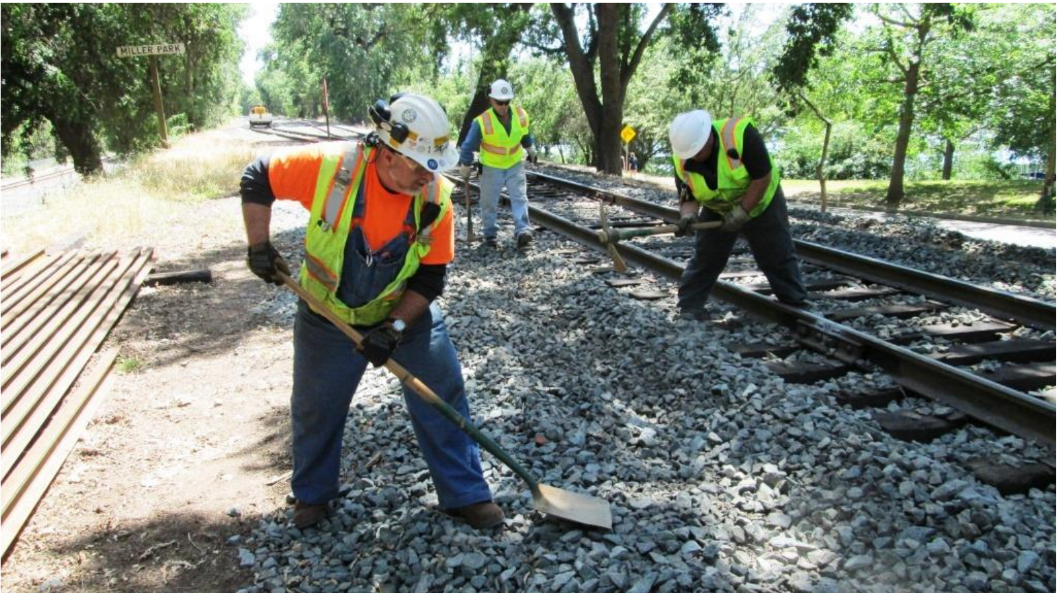
In the afternoon, Mike F., Joe, and Anthony start off clearing a mound of rock left by the ballast regulator during the "incident"...
