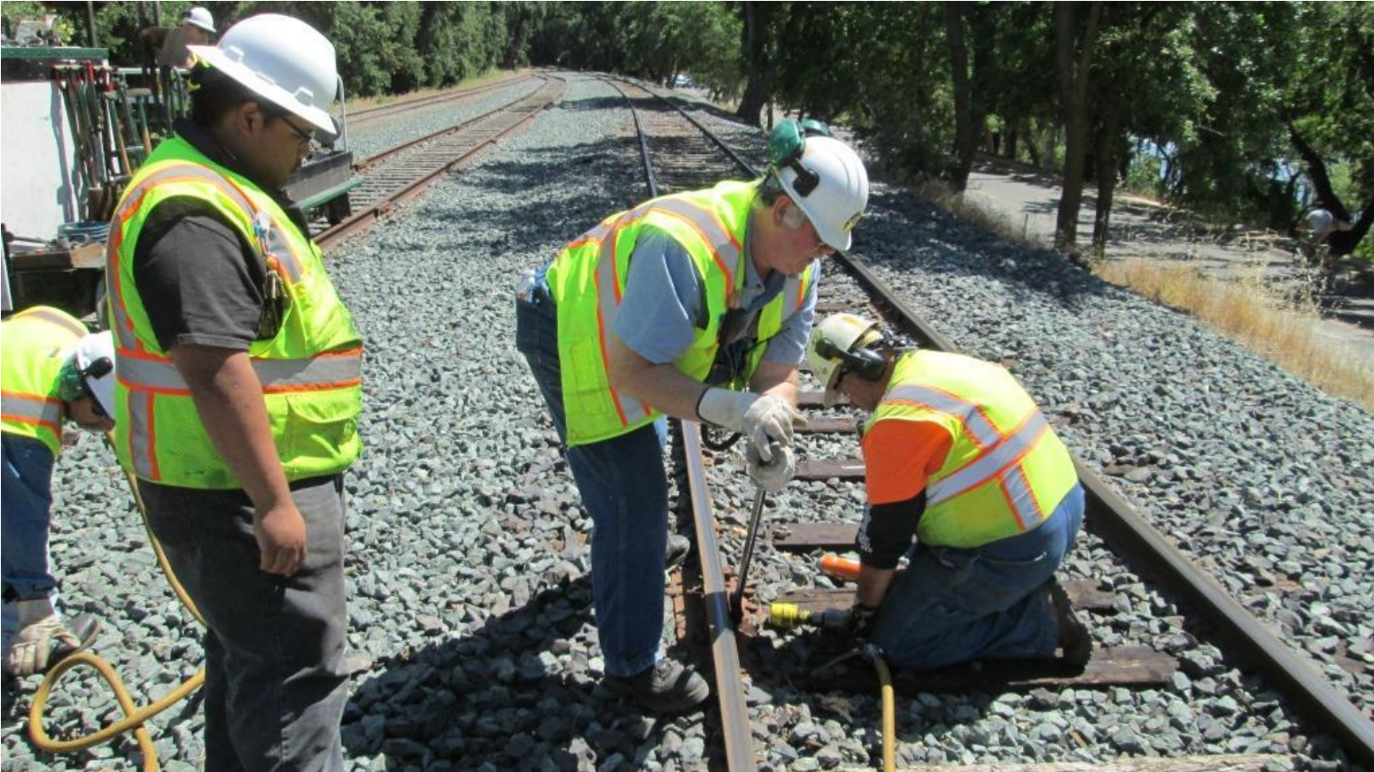
But, when the impact-wrench proved too weak, Chris C. comes in to loosen the nut by hand
