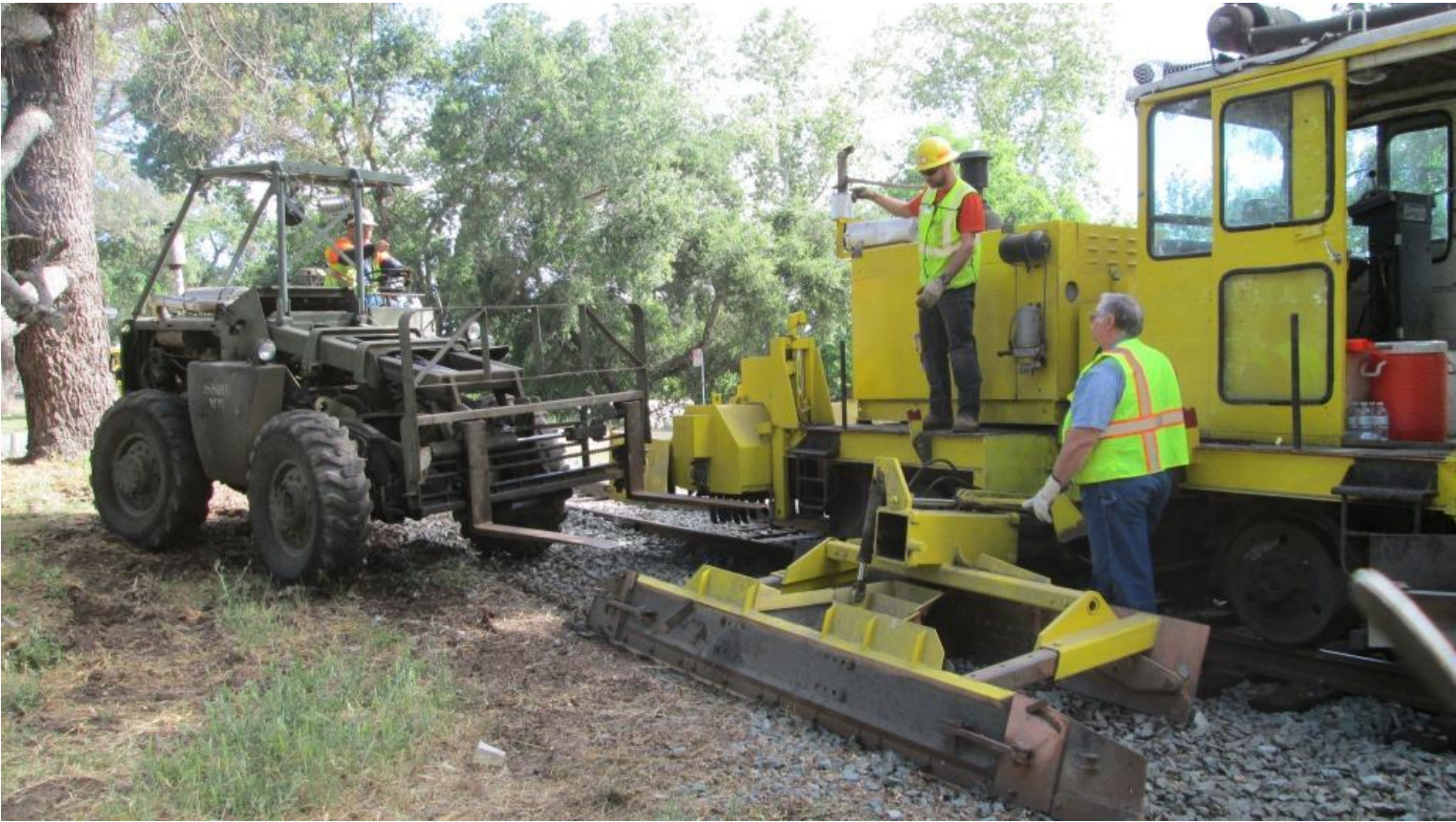
Chris M. provides direction for Mike F. on the Green Machine in straightening out the catawampus wing
