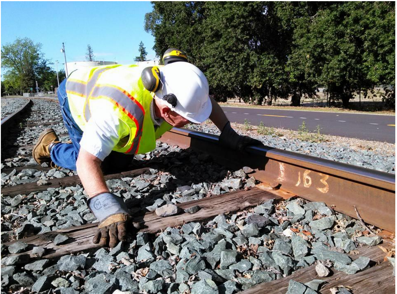
Clem looking for the rail-weight engraving on web of the rail to determine the size of the ratchet needed on the bolt-machine
