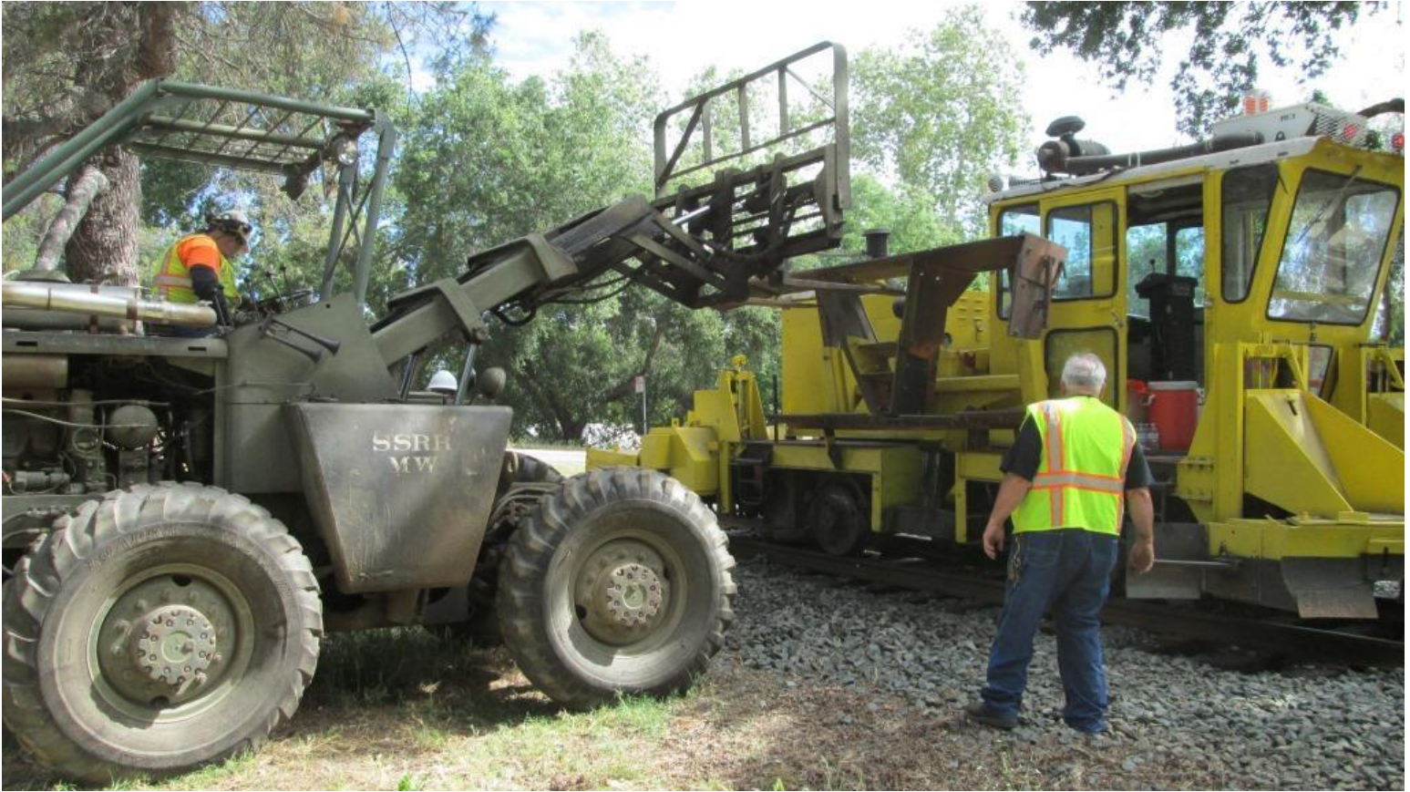
Success! With the wing secured, the regulator can be moved and will not be blocking any trains
