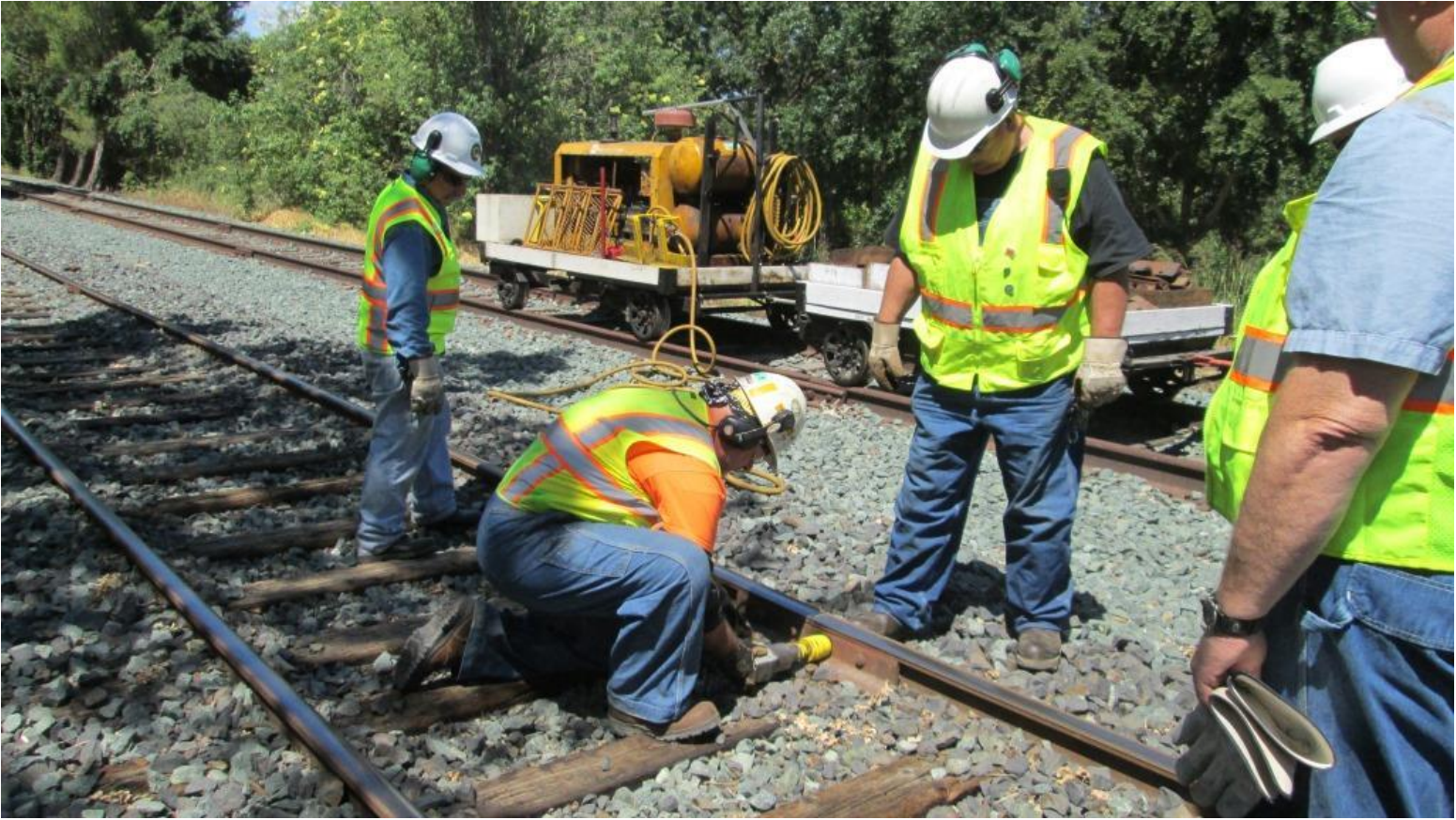
Mike F. uses the impact wrench to remove a nut in order to replace the lock-washer as Harry holds the bolt in place to keep it from spinning
