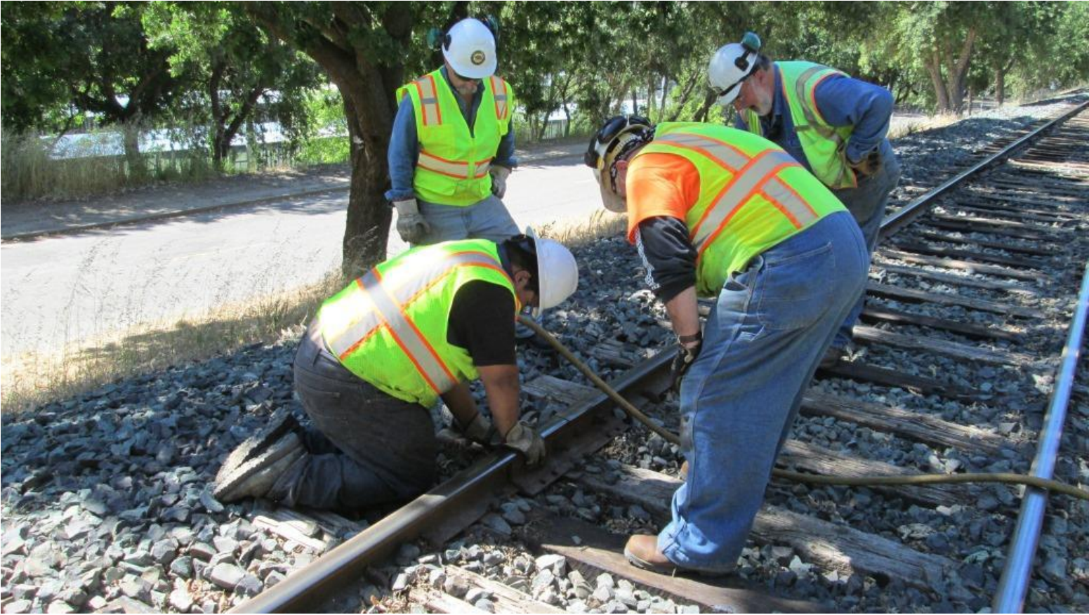
Anthony takes on the next bolt with a broken lock-washer
