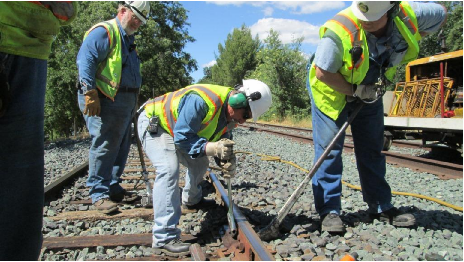
After the nut was split by the track-chisel, Joe removes it the rest of the way while Chris C. uses a claw-bar to hold the bolt from spinning
