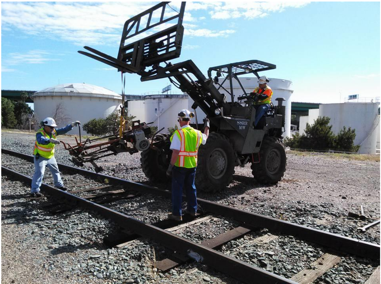
Joe, Clem, and Mike F. deploy the bolt-machine
