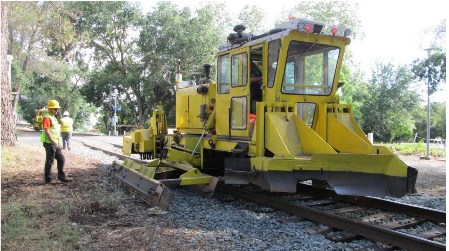
Chris M. provides guidance from the ground as Chris C. operates the regulator
