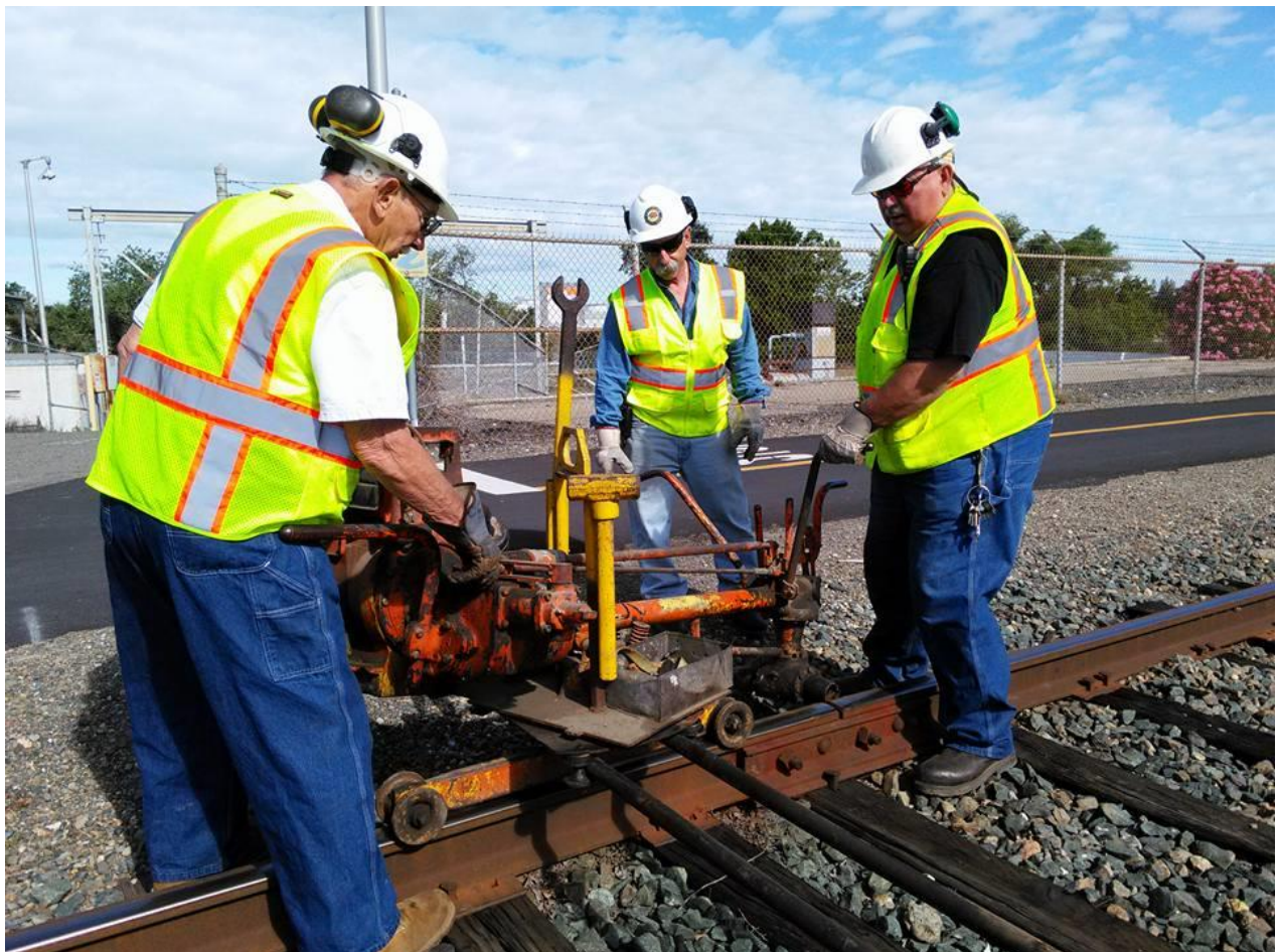
Clem, Joe, and Harry with the bolt machine in action
