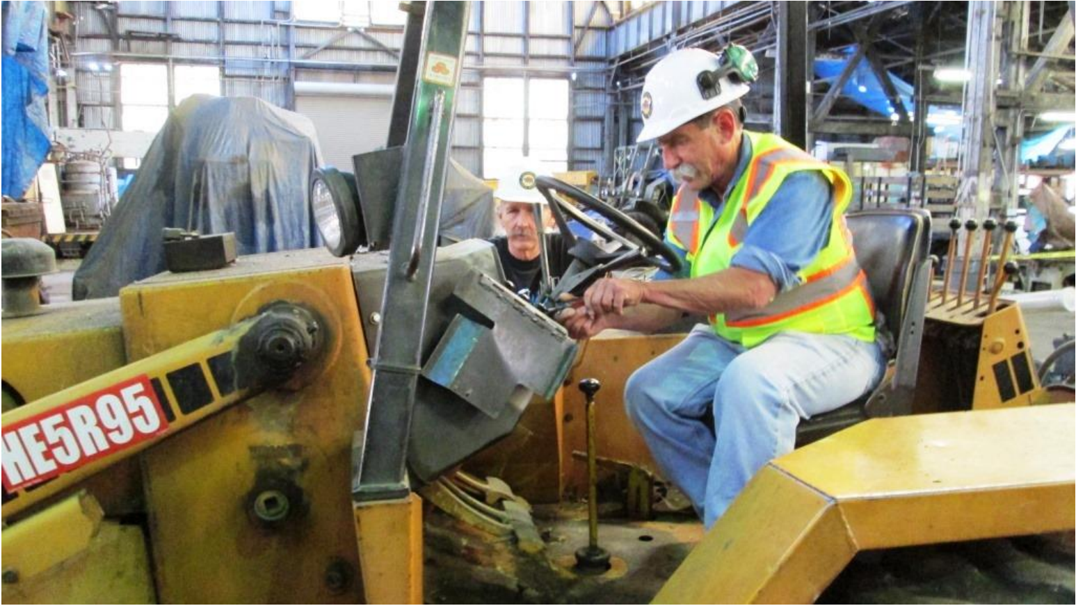
Joe and Fred addressing the electrical issues on the back-hoe
