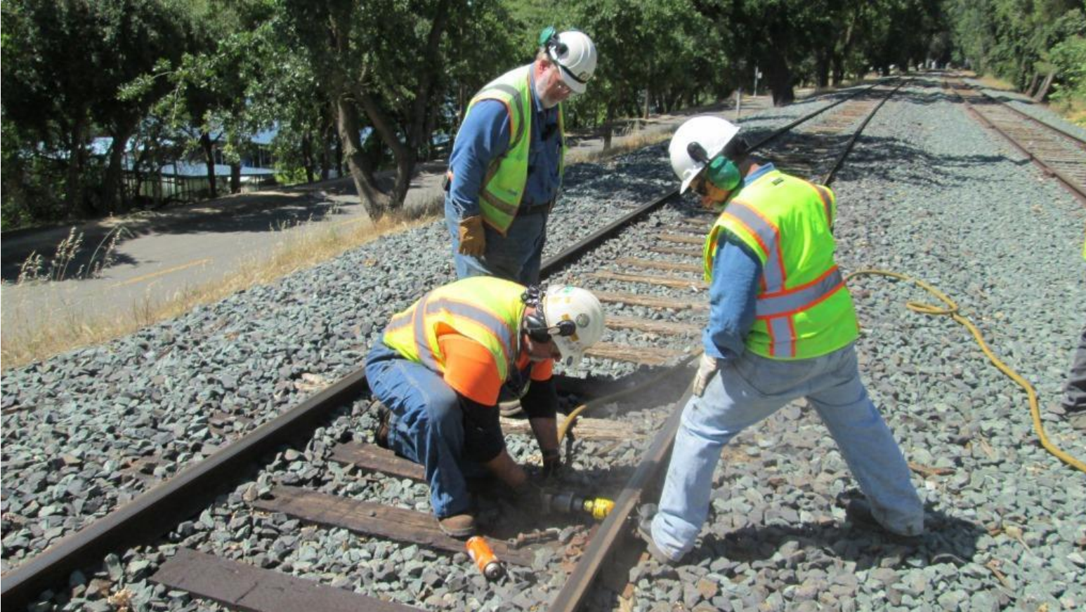
Now Mike F. uses the impact-wrench to tighten down a new bolt
